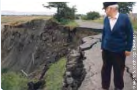
A public road used by school buses falls victim to the greed for more coal in Lanarkshire, Scotland.
